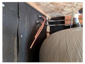
o Close pressure tank drain valve.
