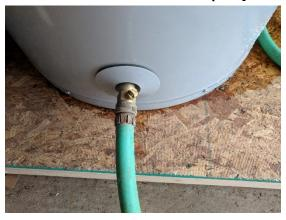
Close settling tank drain valve almost all the way. (Allows the system to flush sediment)
