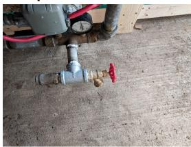
o Close heater drain valve. (Requires a flat head screw driver)
