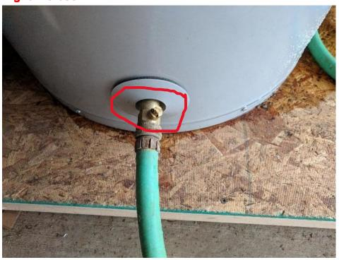
Open settling tank drain valve. Open half way = Handle should be in line with pipe and then bring it back to half open. (Allows the system to flush sediment but not too much pressure)
