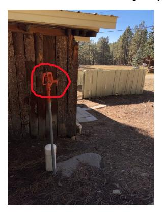
Remove PVC CAP and Turn to On (Open).
